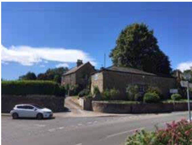
b 'City Square' looking west across Main Street.
